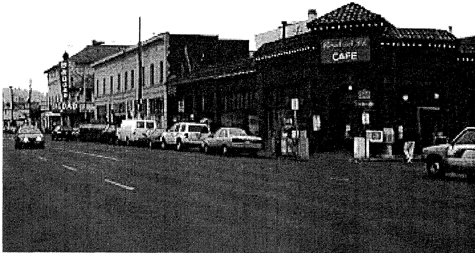
Figure 7. Storefront Commercial Development along SE Hawthorne.
