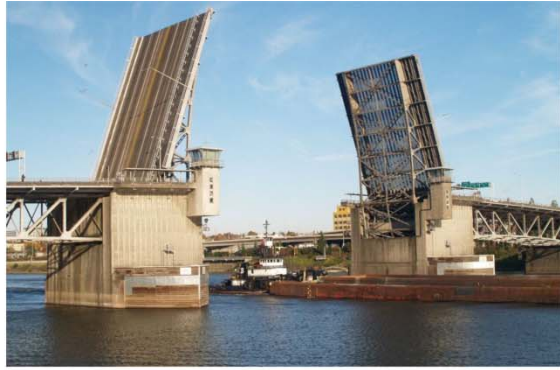
(b) Morrison Bridge with lift span up
