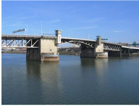
(a) Morrison Bridge with lift span down
