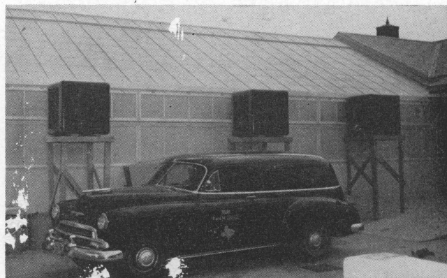
Figure 1. Installation showing use of conventional evaporative cooler.
