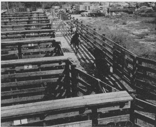
Figure 4. Delivery alley at new truck cattle docks.
