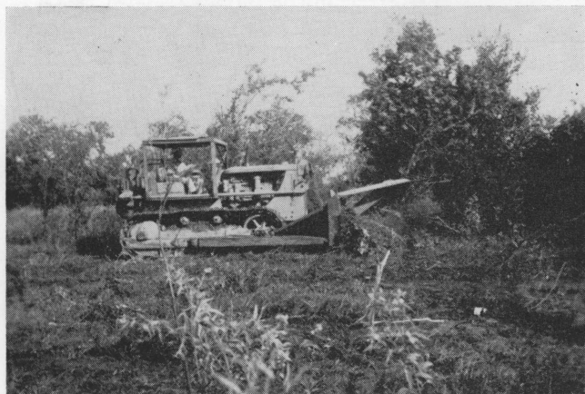
Figure 3. Bulldozing is relatively effective in clearing oak and cedar.
