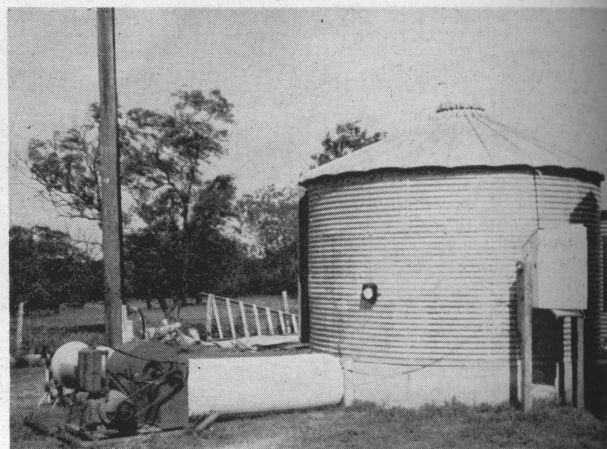
Figure 7. This bin had a false floor and was used for drying flaxseed with heated air.
