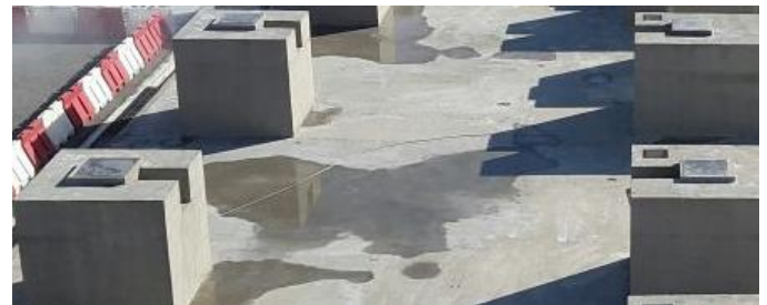
Figure 24: Onshore Module Aboveground Foundation Detail
