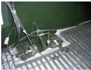
Figure 8: Accelerometers installation on LCC foot
