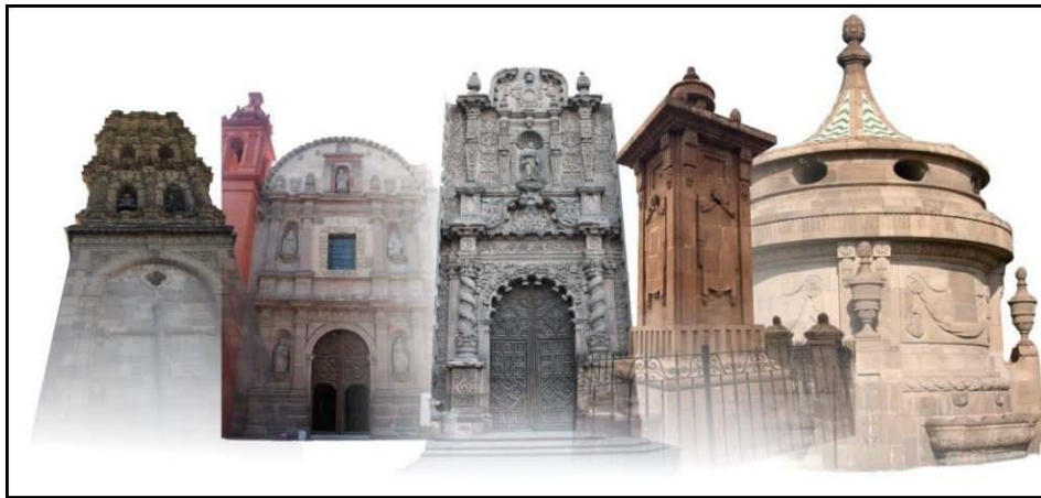
Fig. 1: Some of the principal buildings and monuments build with the Cantera Rosa. Left to right: Tower and facade of the San Agustín Church, facade of the El Carmen Church, fountain in the Santuario and Santuario del Desierto Church.
