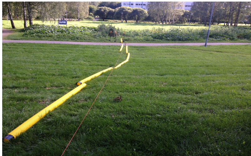
Figure 3.1 Protective pipe I dug into the ground to contain the electrical cables that connected electricity from a neighbouring house to the sound installation.
