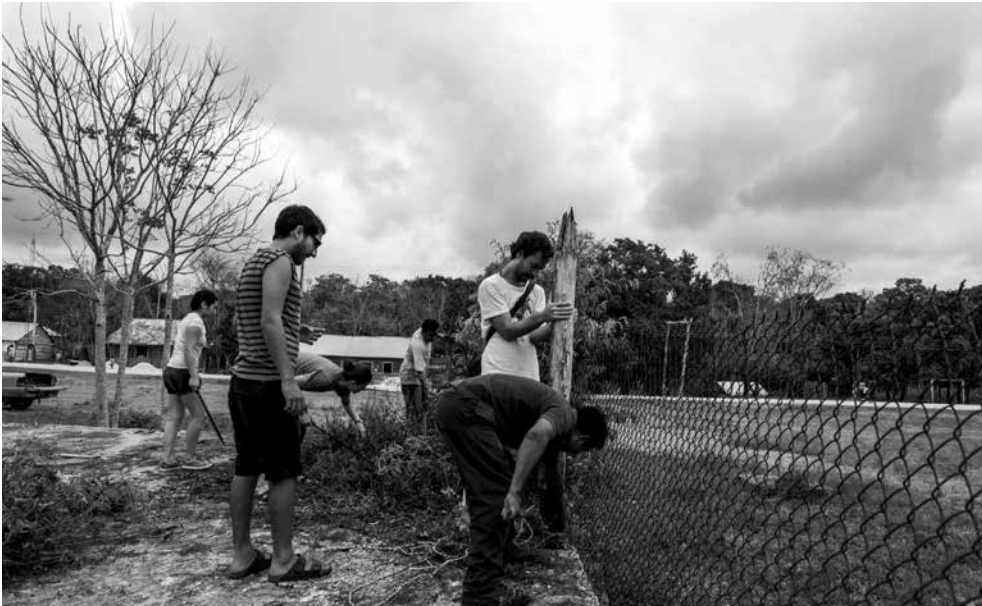
Figure 86. Everyone cleaning the construction site. Photo by Jan Ahlstedt.
