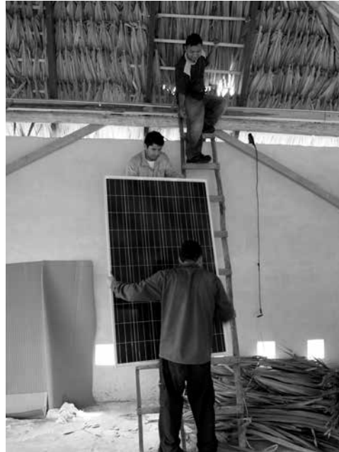
Figure 93. Rodolfo and Raúl (Yéclabuilti), and Rogelio (El 20), installing the solar panel on a base that Sayuri, Miriam and I made at their workshop. Picture by Claudia Garduño.
