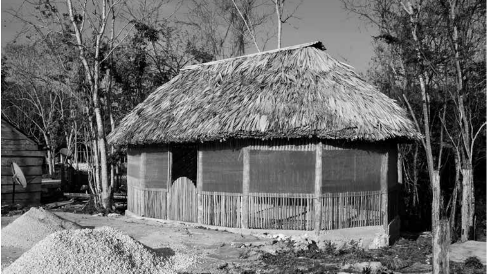
Figure 81. Construction sponsored by Pronatura, and built by the ejidatarios of El 20 through 'fajinas'. Photo by Jan Ahlstedt.
