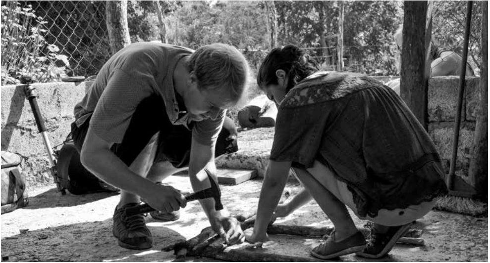
Figure 54. Isela and Ismo building a rack for placing bottles and using UV light to kill microorganisms. Photo by Jan Ahlstedt.
