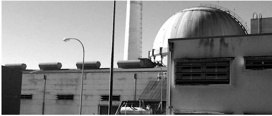
Figure 8.9 The José Cabrera Nuclear Power Station.
