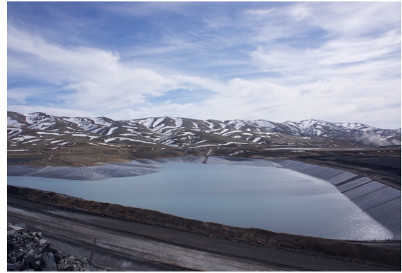
(b) Terrestrial view of a tailing pond in Elko, Nevada.
