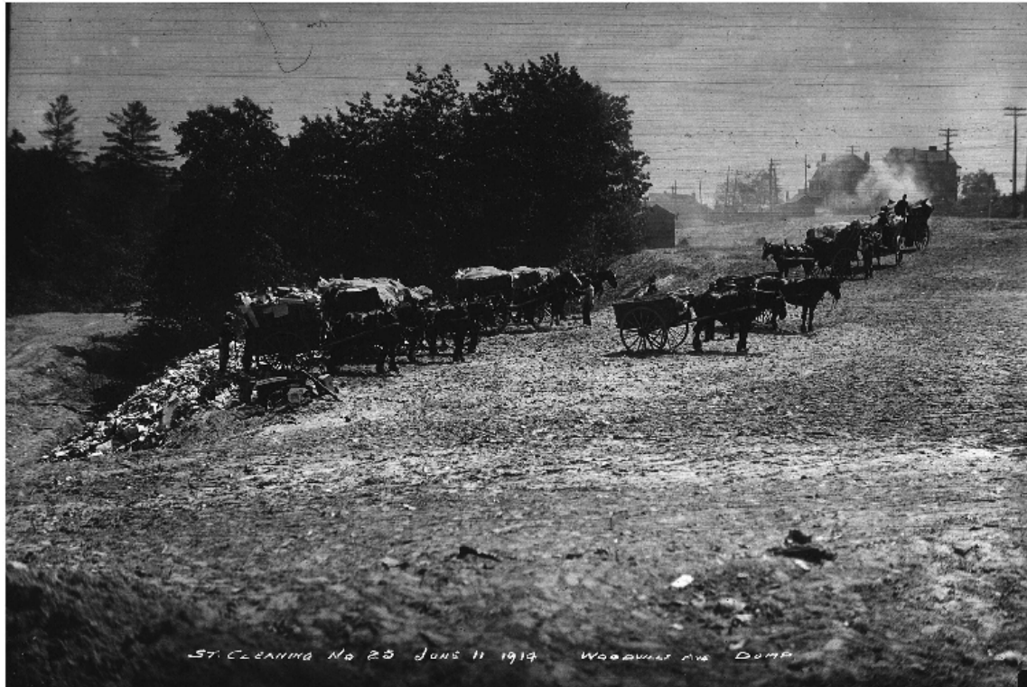
Figure 3.3 “Woodville Avenue Dump”, June 11, 1914. City of Toronto Archives, Fonds 200, Series 372, Sub-series 70, Item 25. As can be seen, wastes were still predominantly transported by horse and wagon to these ravine fills/open dumps.
