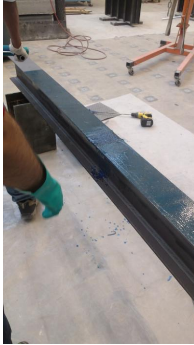
Saturation of base layer prior to applying longitudinal fabrics
