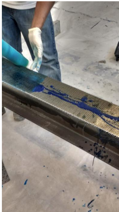
Application of longitudinal fabrics
