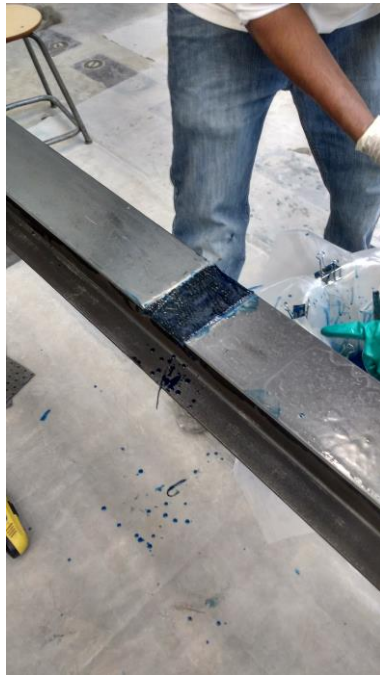
Application of small fabric pieces to corrosion gap
