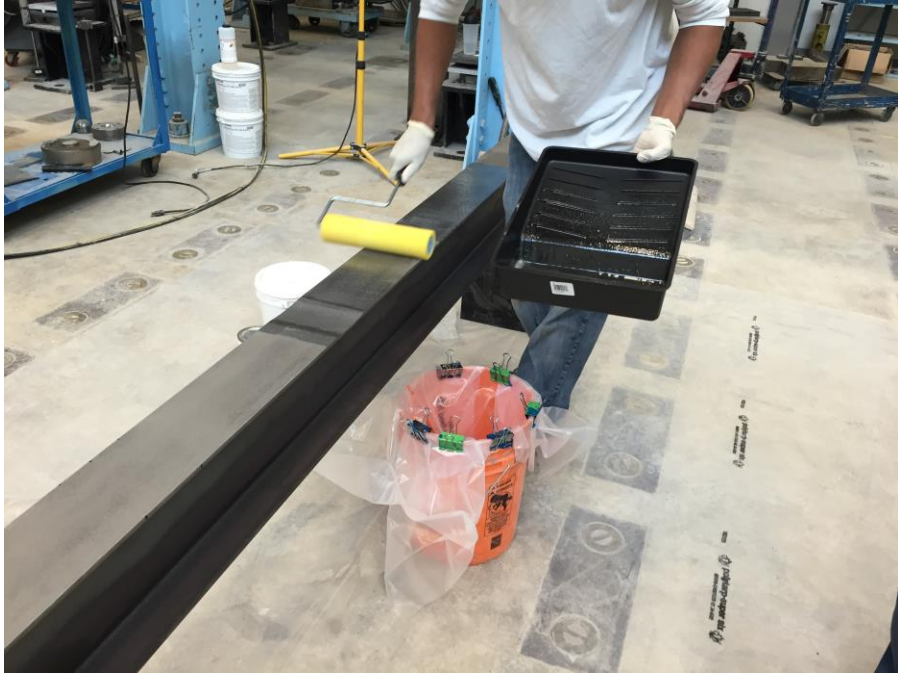
Application of primer to sandblasted beam
