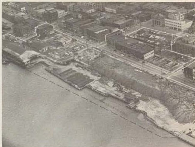
An unsightly mixture of commercial and industrial buildings characterized the riverfront at the foot of Ouellette Ave.
