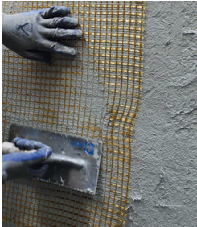
Figure 1.7 Application of FRCM (adapted from Ruredil )
