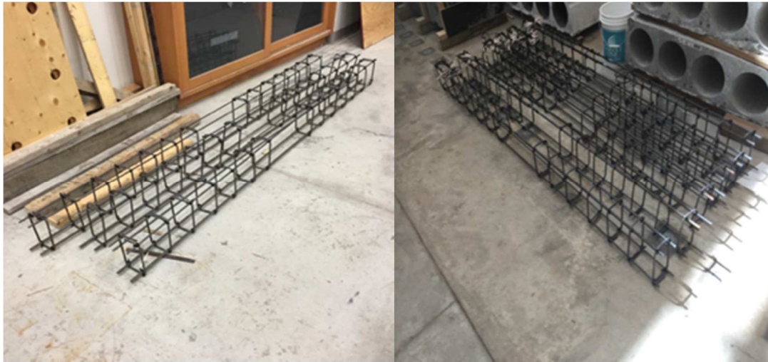
Figure 3.8 Fabrication of steel-cages for RC beams.
