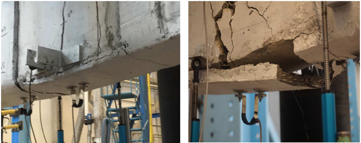
Figure 4.20 Glass-FRCM strengthened beam, A4-G-4L, failure mode
