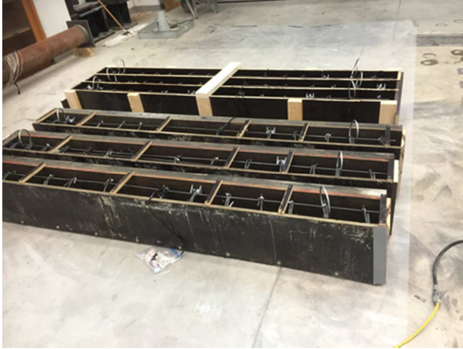
Figure 3.7 Formwork for fabrication of RC beams
