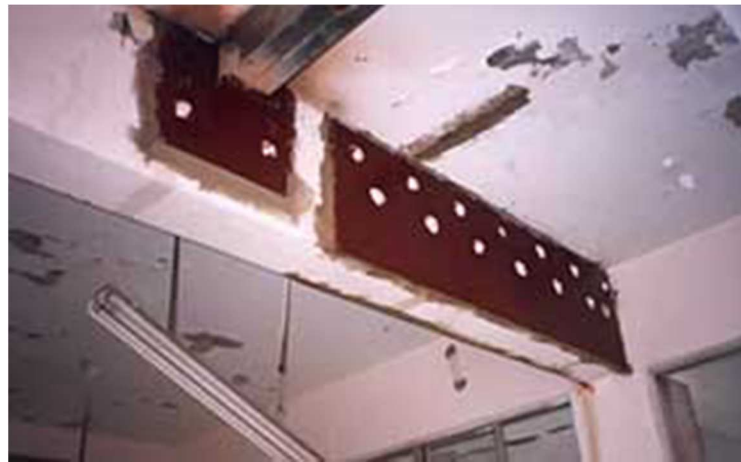
Figure 1.2 Steel plate bonding (adapted from chemosystems )
