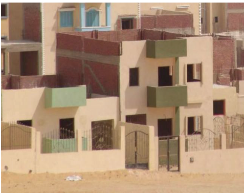
Step 5: Second Floor Completed with External Finishings
