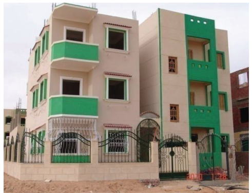
Step 6: Three-Floor Building Completed with External Finishings
