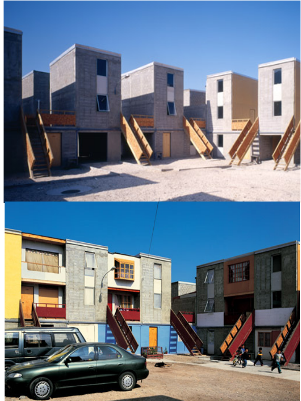
Figure 3: Evolution of the core unit in Quinta Monroy, Santiago de Chile before the expansion (above) and after (below) (Photo: Universidad Católica de Chile, 2012)
