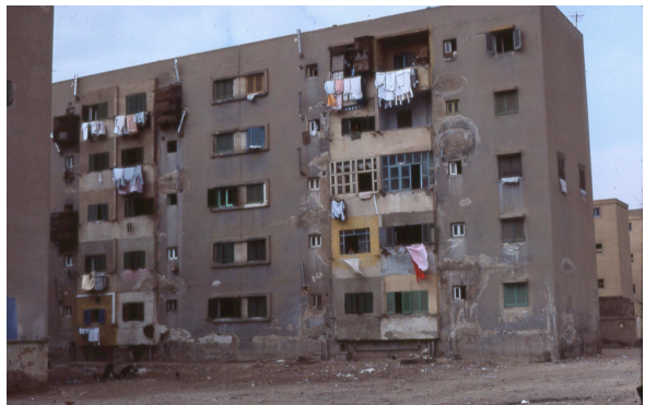
Figure 2: Example for the deteriorated conditions found in 1983
