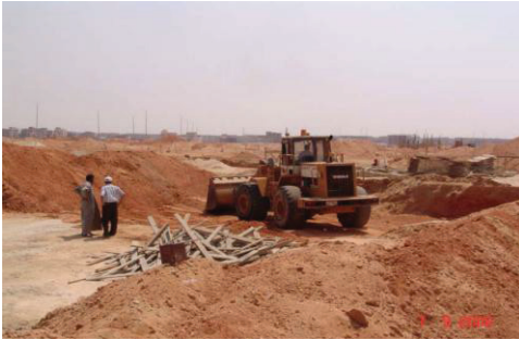
Step 1: Land Preparation and Excavation
