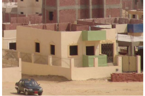
Step 4: Ground Floor Completed with External Finishings
