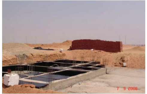
Step 2: Building Foundations
