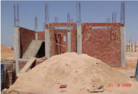
Step 3: Ground Floor Columns and Walls
