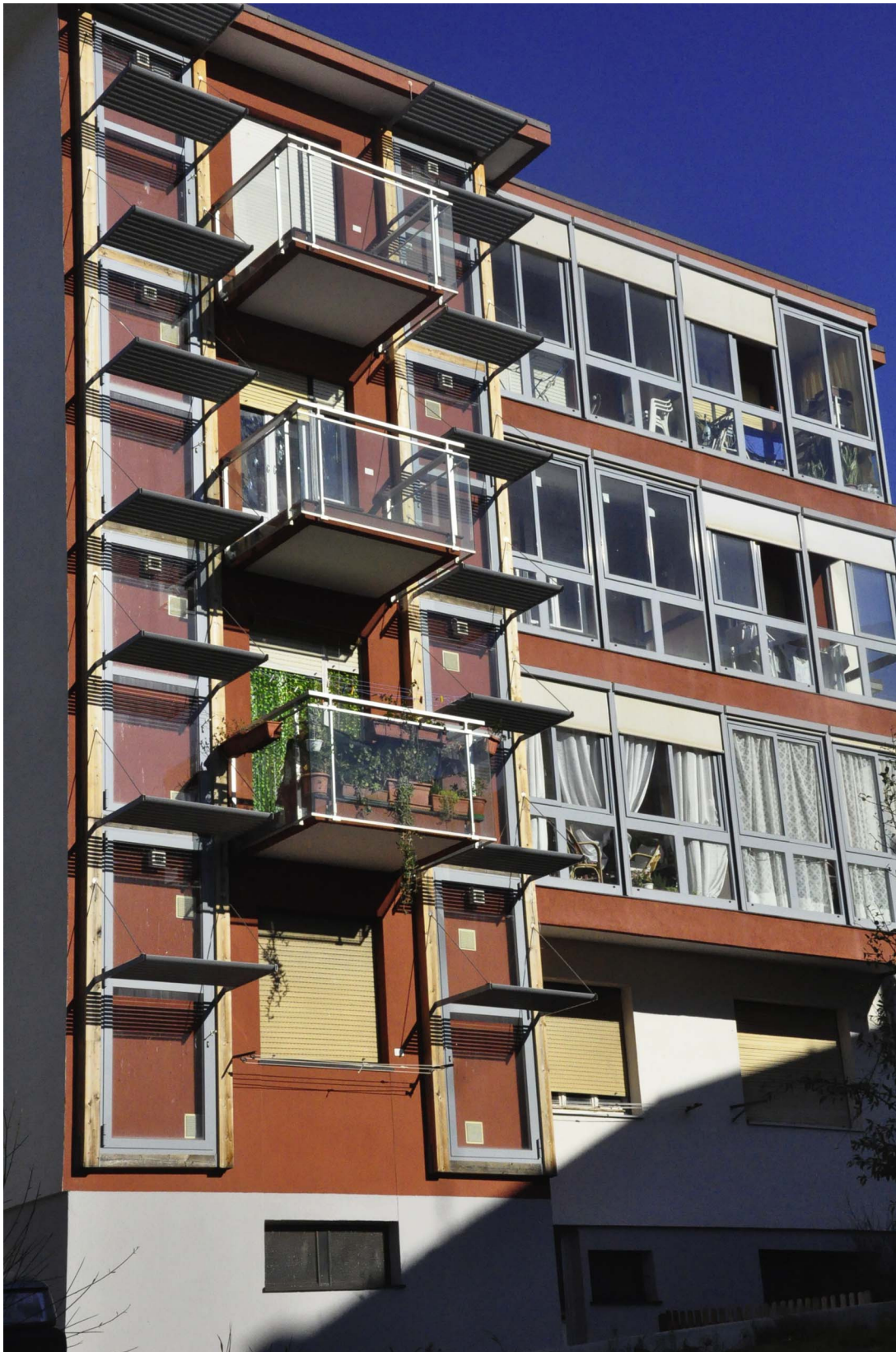
Fig. 3. Building C, South Façade with Solar Greenhouses and Trobe-Michel walls.
