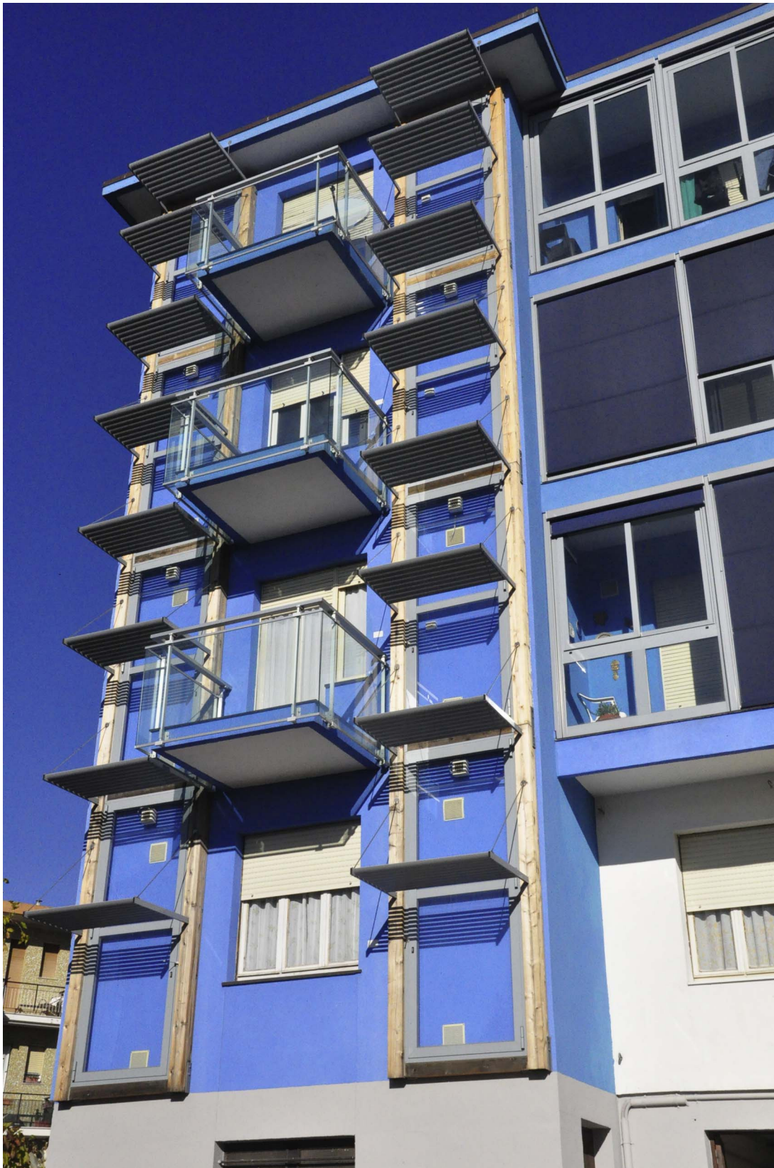
Fig. 2. Building B, South Façade with Solar Greenhouses and Trobe-Michel walls.
