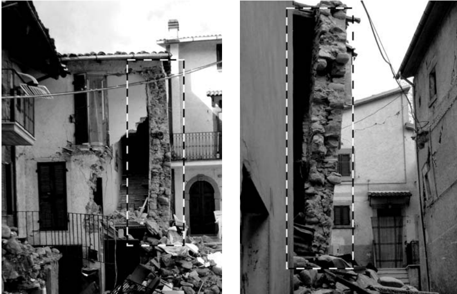
Figure 9 Double wythe masonry wall (Accumoli)
