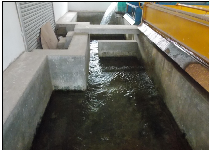
Figure 3.5: Downstream Volumetric Tank
