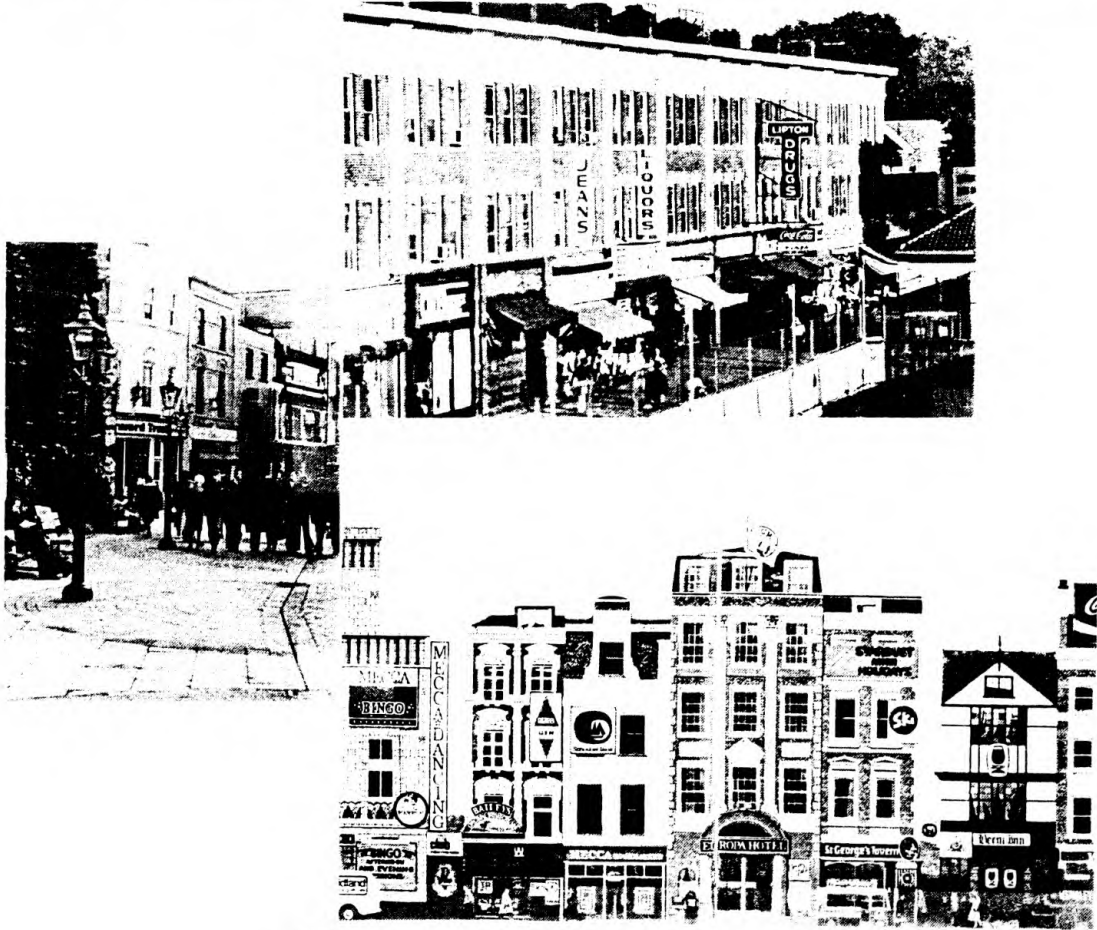
Figure 9.9: Before and After Images of Facade
