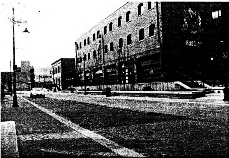
Figure 3.13: South End of Mosley Street
