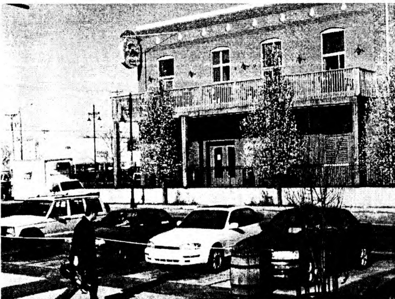
Figure 3.14: River City Brewery Adjoining Mosley Street
