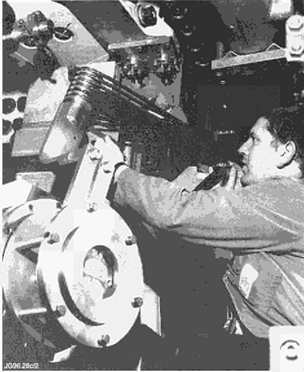
Fig.74: Installation of Vessel Supports:
