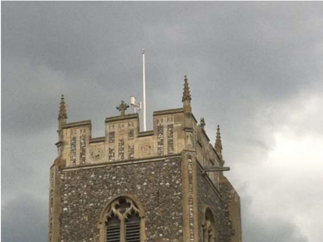
Figure 6: WiSpire repeater mast, Holy Trinity Church, Loddon. Source: Author.
