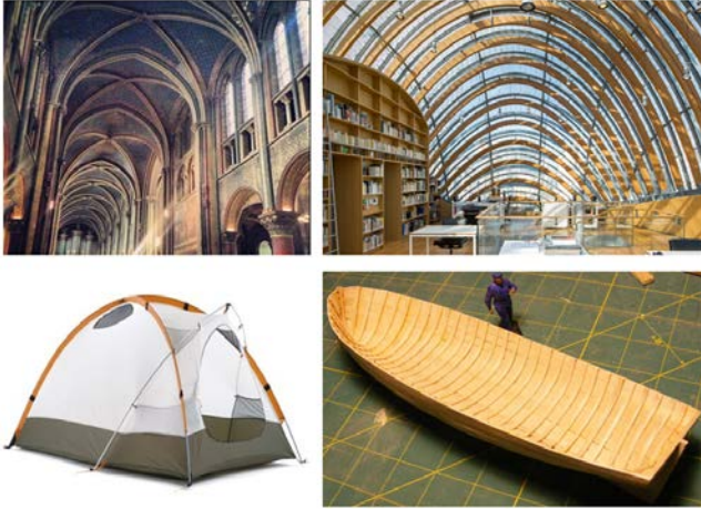
Figure 2: Various forms of rib-reinforced shell structures. Top left: rib vaulting in the nave of Reims Cathedral. Top right: transparent bubble dome with ribs of larch. Bottom left: a tent. Bottom right: a boat.
