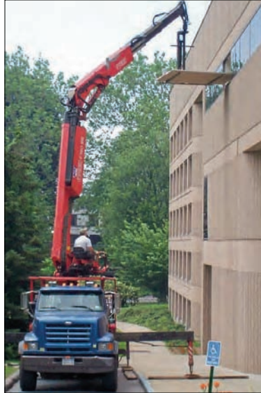
Sheetrock and cement delivered via crane through window in Glass Building
