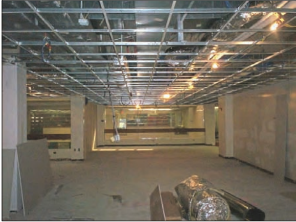
The grid for the ceiling tiles is installed
