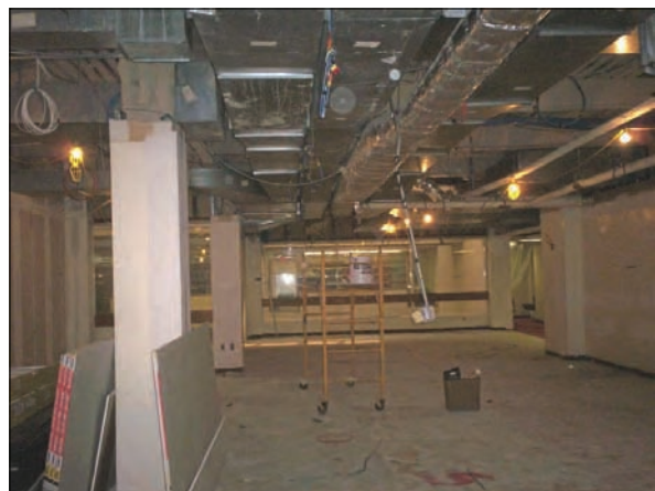
Wiring (electrical and network) and ductwork for heating and cooling
