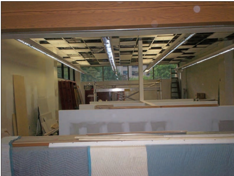
September: installation of the new Circulation Desk
