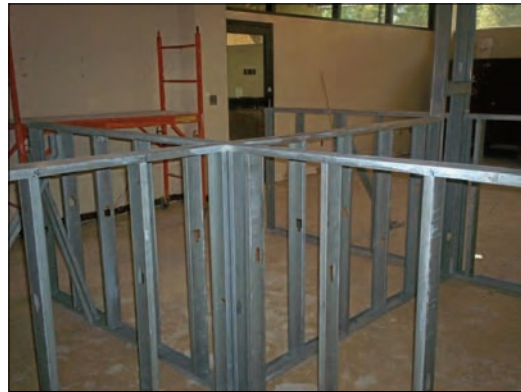
Framing for new staff areas behind circulation
