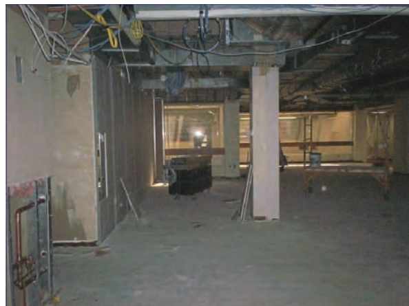
Electrical and network wiring, and more drywall
