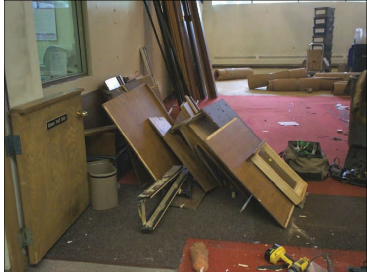
August: Demolition work begins in the Circulation area
