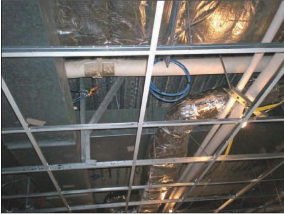
The grid for the ceiling tiles is installed
