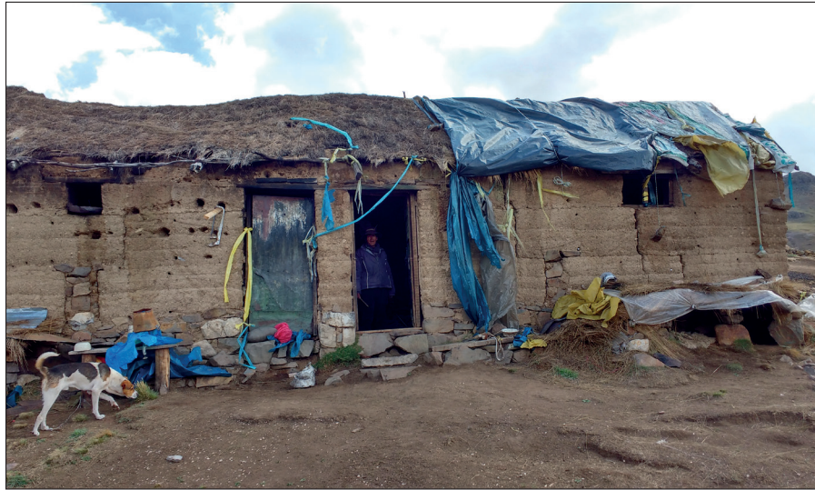
Image 10. Homes are makeshift structures made from rudimentary local materials like stone, mudcap and wood.
