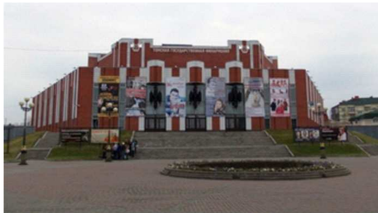
Figure 3. The building of the grand concert hall of Tomsk city
