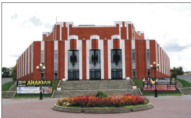
Figure10. The building of the grand concert hall of Tomsk city with the proposed promotional displays.
