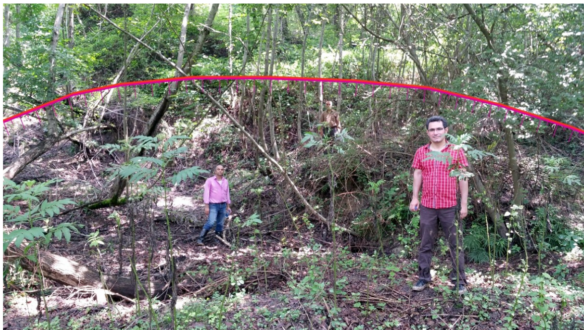
Figure 7. Ground picture of one of the scarps (red line) observed in the landslide detected by ALOS data analysis
