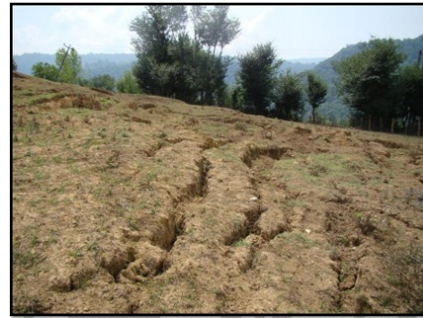
Figure 2: A landslide-prone area with tensile cracks in the northwest-southeast direction
