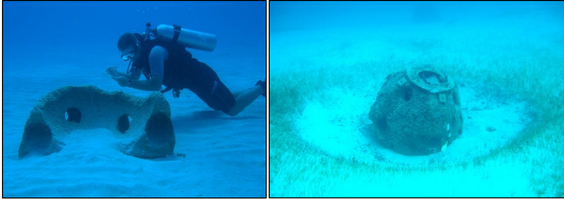
Figure 2.16 Hydrodynamic effects from Hurricane Dean on SM deployment field: left) fragments of a broken module in Akumal, and right) scouring around the base of a module in Puerto Morelos.
