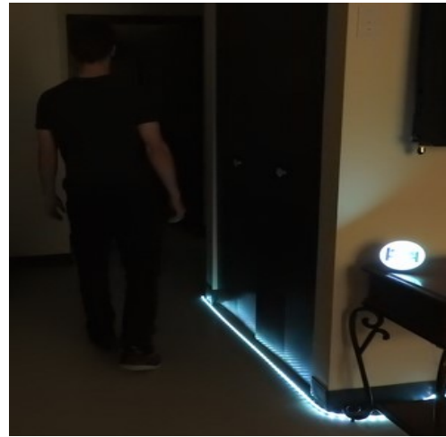
Figure 33. Visual indicator and light path for accompanying the person to the room.
