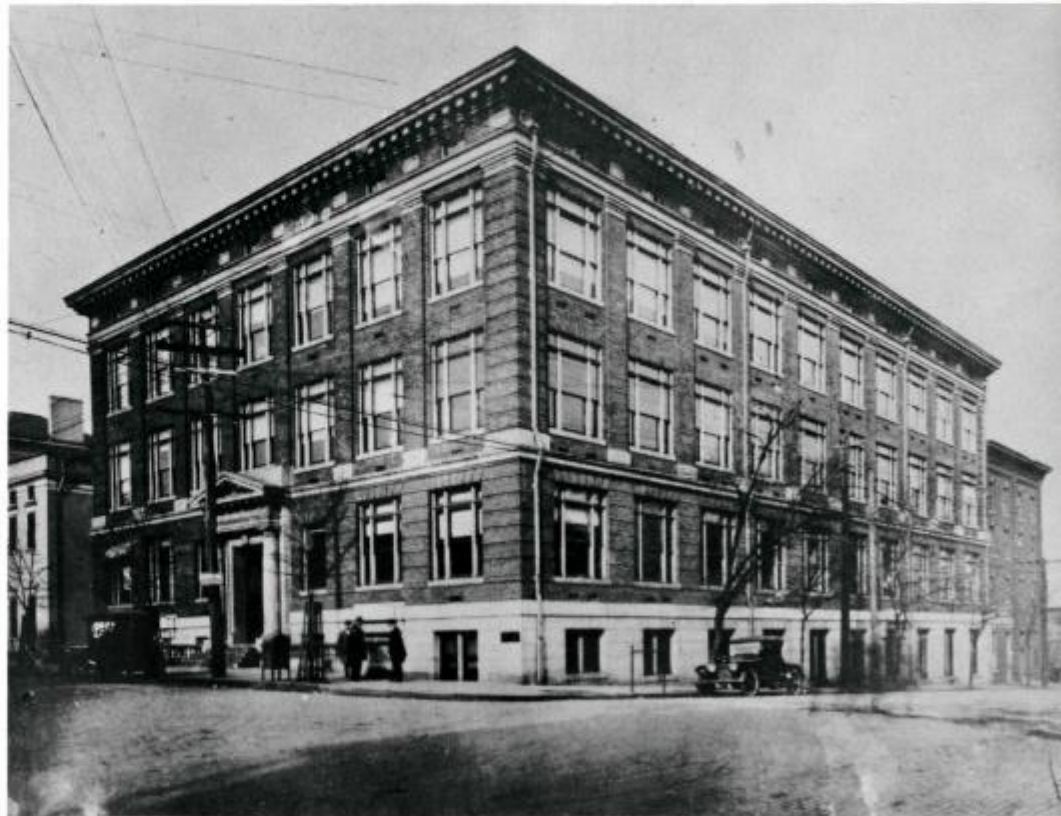
McGUIRE HALL as it was when consolidation was effected in 1913. Built in 1912 by University College of Medicine at a cost of $208,053, it is named for Dr. Hunter Holmes McGuire. During the session 1940-1941, a fourth story was added at a cost of $150,000.
