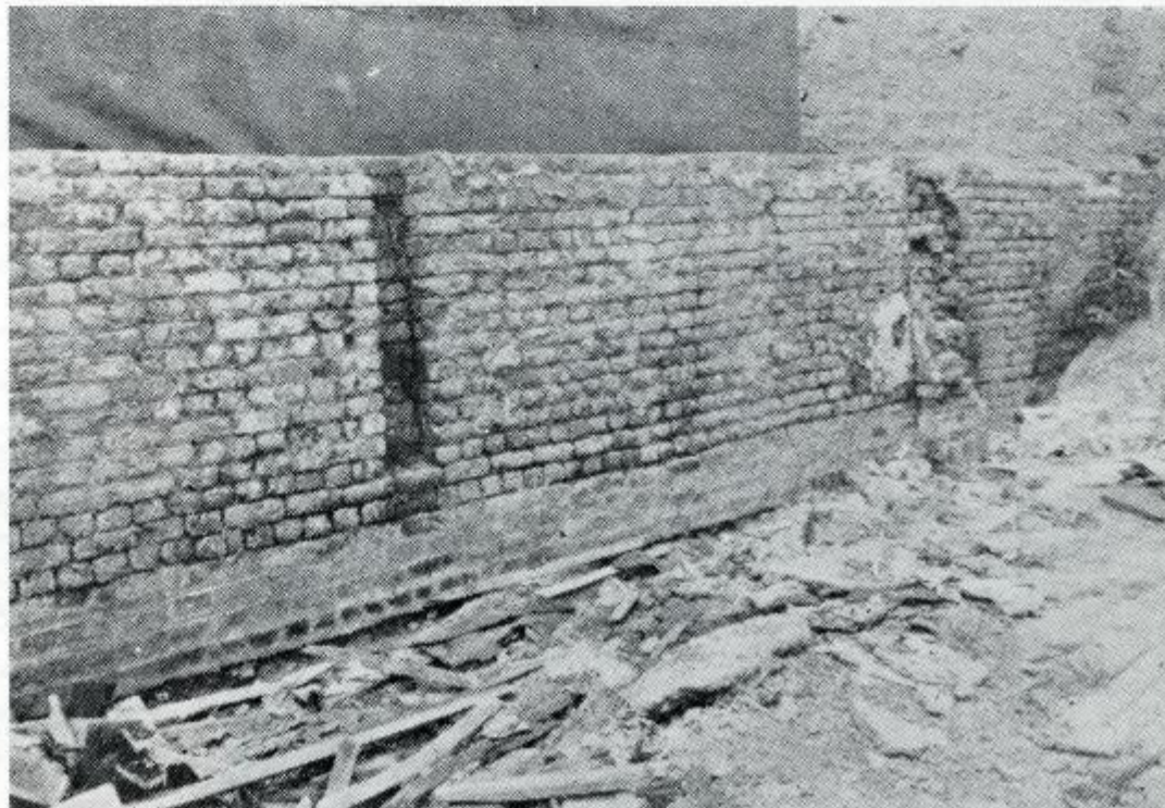
PART OF AN OLD WALL Running along Twelfth Street was excavated in 1938 during construction of the A. D. Williams Memorial Clinic.
