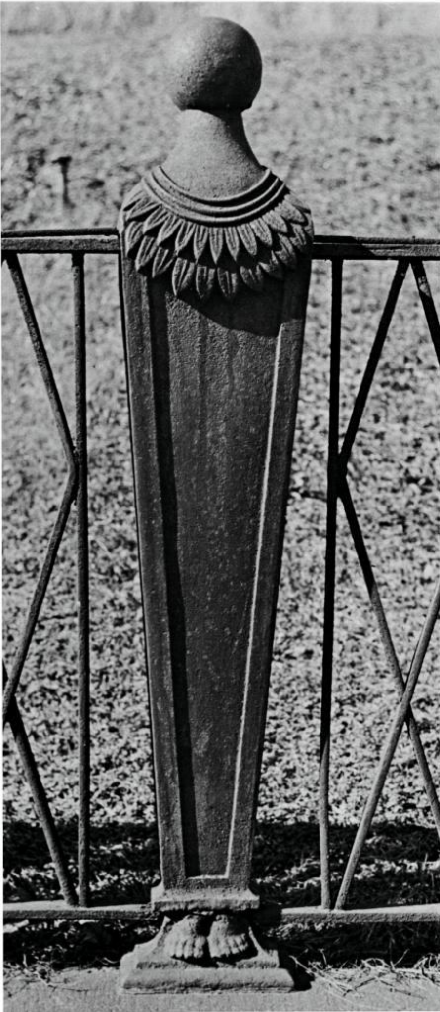
ONE OF THE MUMMY POSTS in the original iron fence, which still guards the building.
