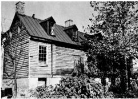
RAZED TO MAKE WAY for construction of Randolph-Minor Hall, this old building was once the home of Jackson B. Wood, father of Dr. Jud B. Wood.
