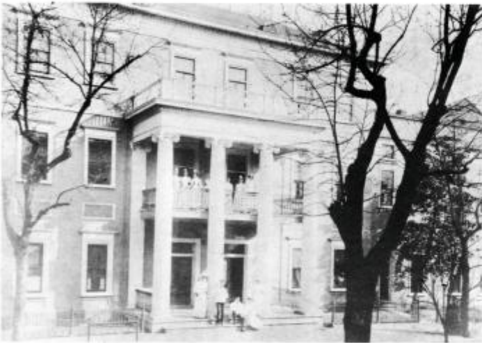
VIRGINIA HOSPITAL about 1900, after a third floor and the columned portico were added.
