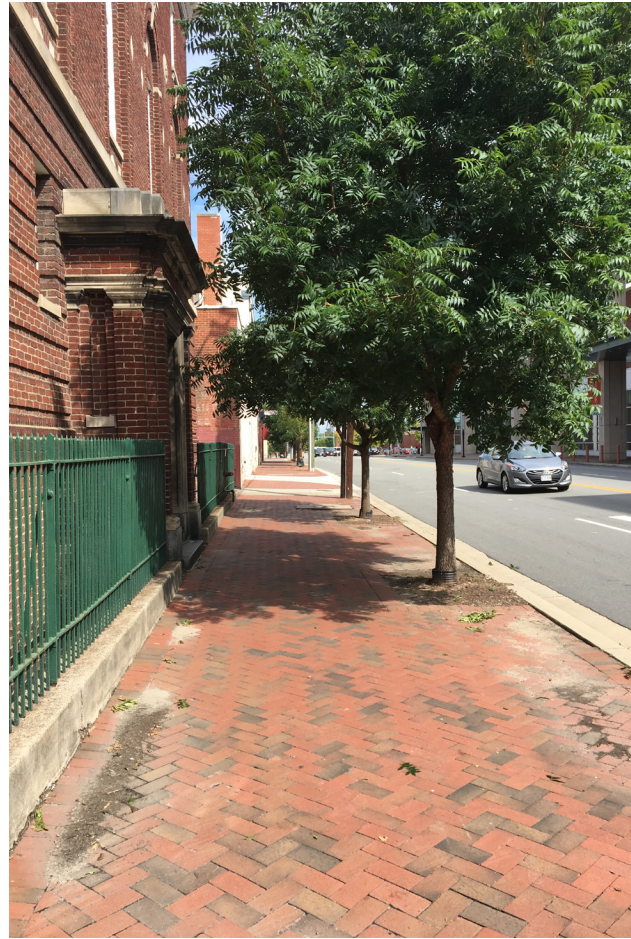
brick pavement leading up to Bliley's Garage
