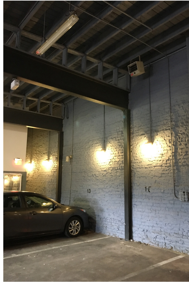
view from the garage: painted brick and the layers of exposed ceiling are visible
