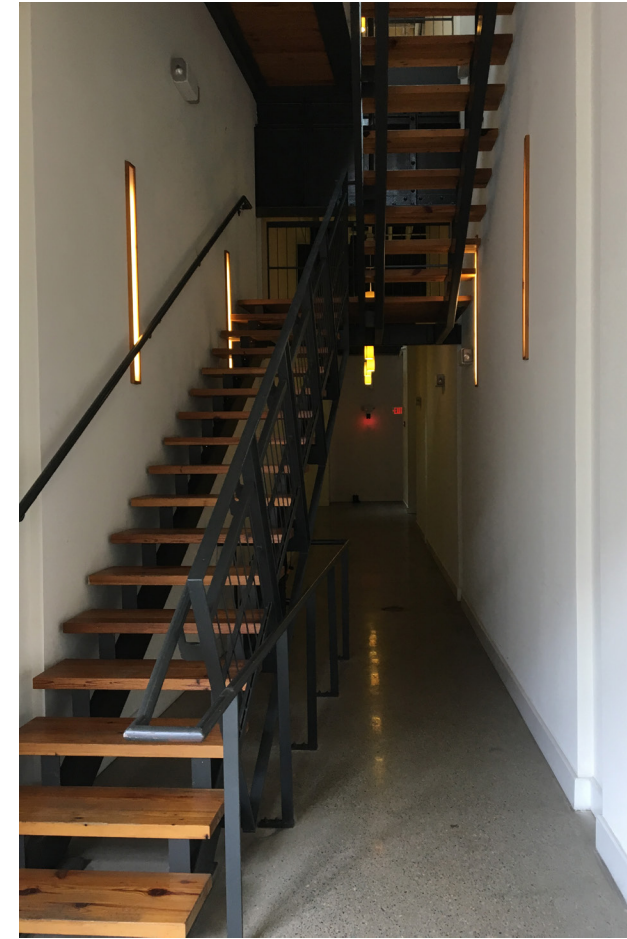
view looking in from front entrance: terrazzo flooring is used throughout the first floor
