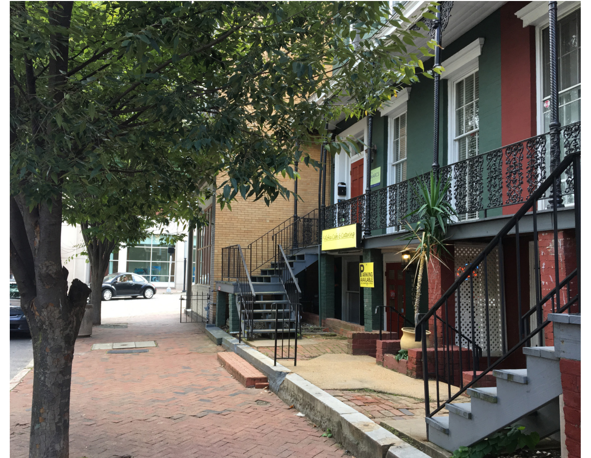
residences located on the same block of n 3rd street
