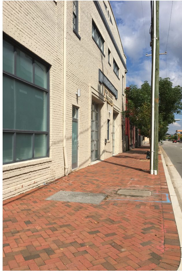
brick pavement sidewalk runs parallel to the facade
