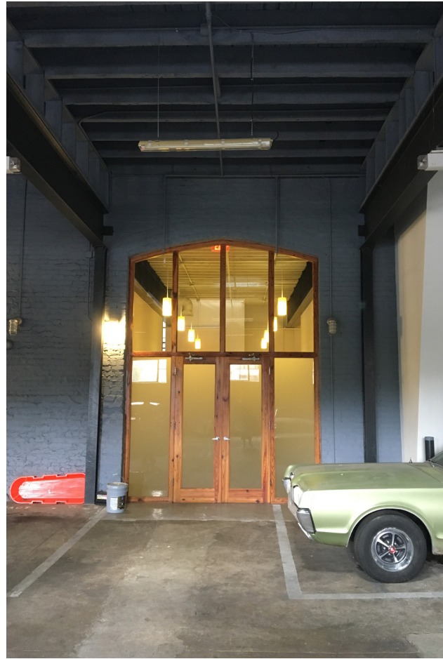
view from the garage: concrete floors and exposed steel beams are evident
