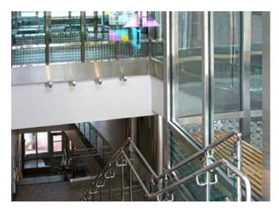
Products such as SuperLite II-XL can be used to form glazing assemblies for fire exit enclosures, such as this one at a St. Cloud University stairway in Minnesota, Source: SaftiFirst.
