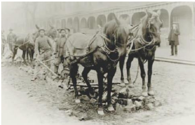
Figure 10: Black laborers plowing cobblestone for construction of the new trolley line. (From the Valentine Richmond History Center as published in Race, Class and Power in the Building of Richmond, 1870-1920 , p. 66)
