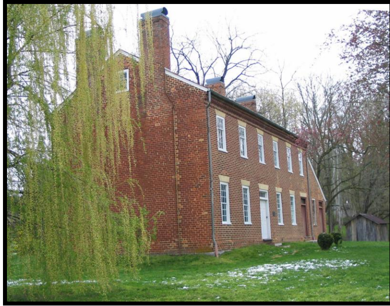
Figure 1. The Doak House Museum. Facing northeast.
