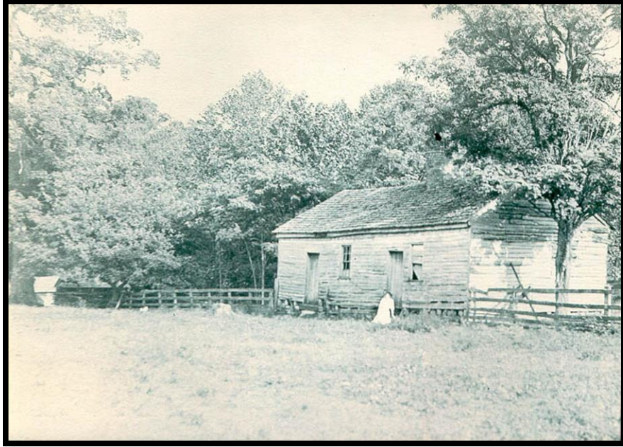
Figure 9. Doak Academy and Springhouse. Undated photograph, facing southeast.
