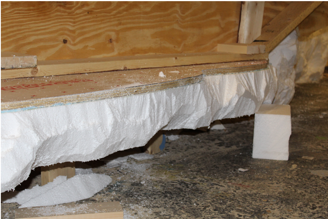
Figure 20: Cut Out Deck Cover with Foam Added and Carved
