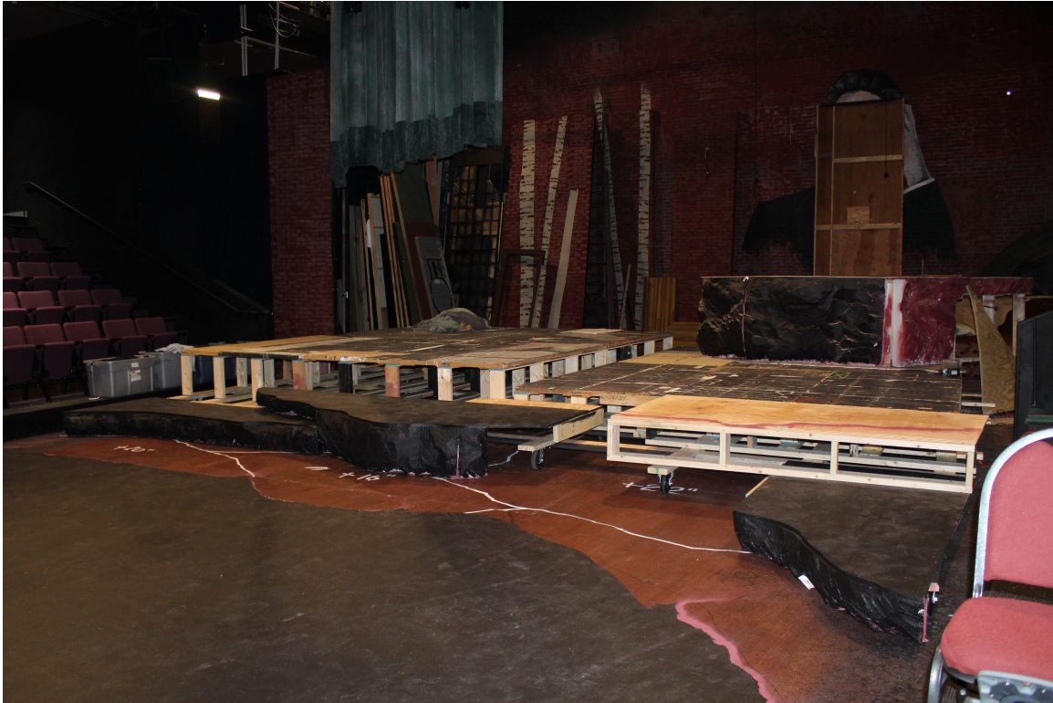
Figure 25: Surface Primer, Foam 2 nd Layer Treatment Viewed from House Left
