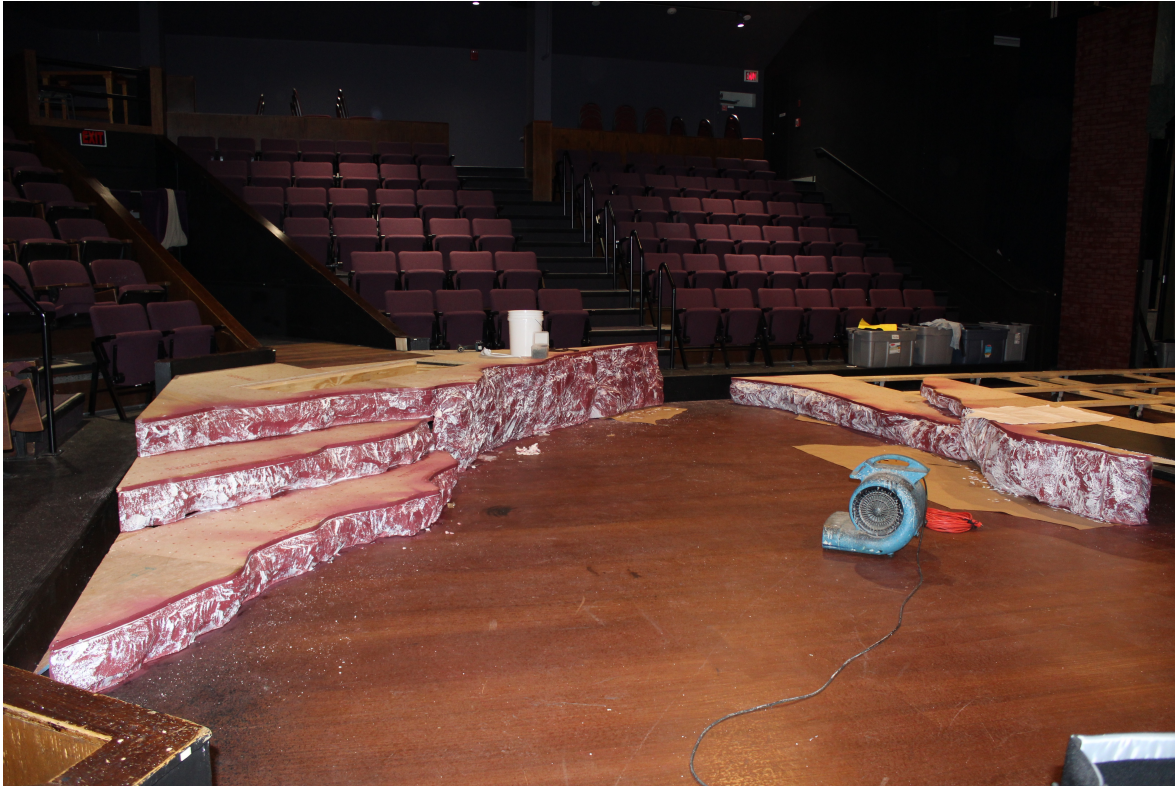
Figure 23: Foam Primer and 1 st Layer Treatment on Downstage Right Vom
