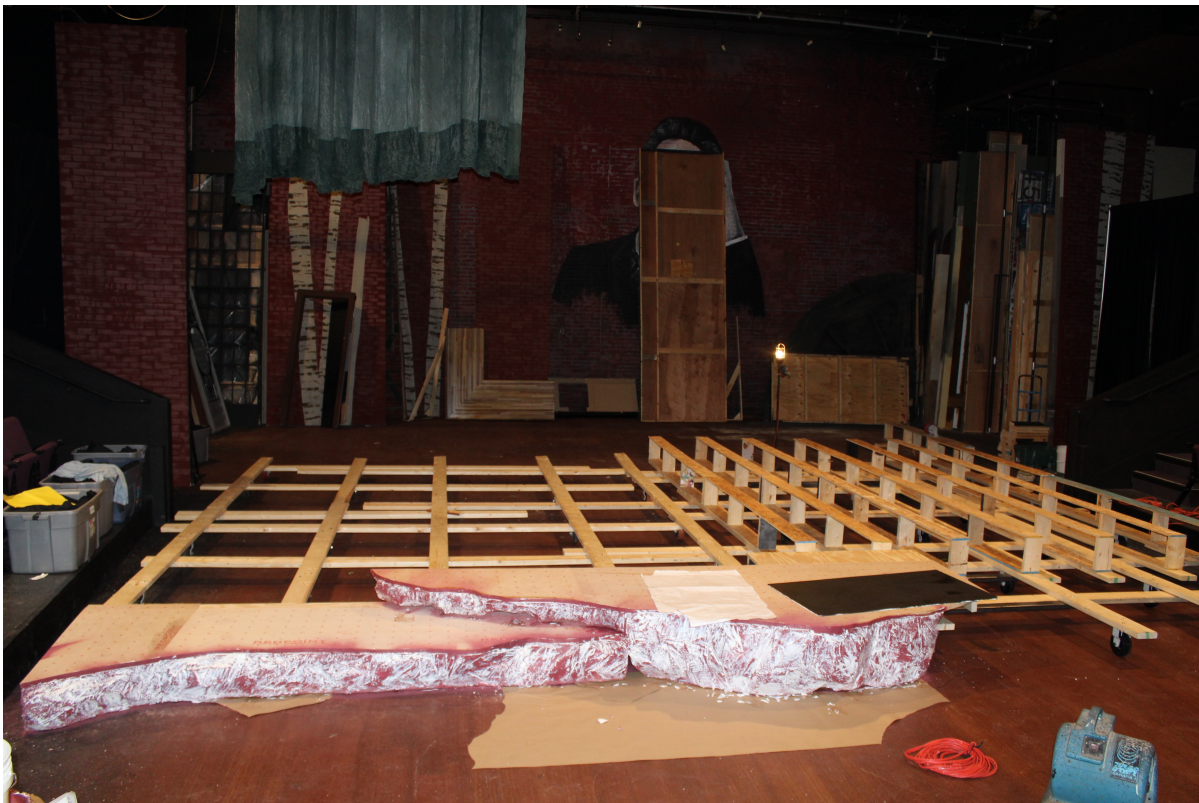
Figure 24: Foam Primer and 1 st Layer Treatment on +8" and +16" Platforms
