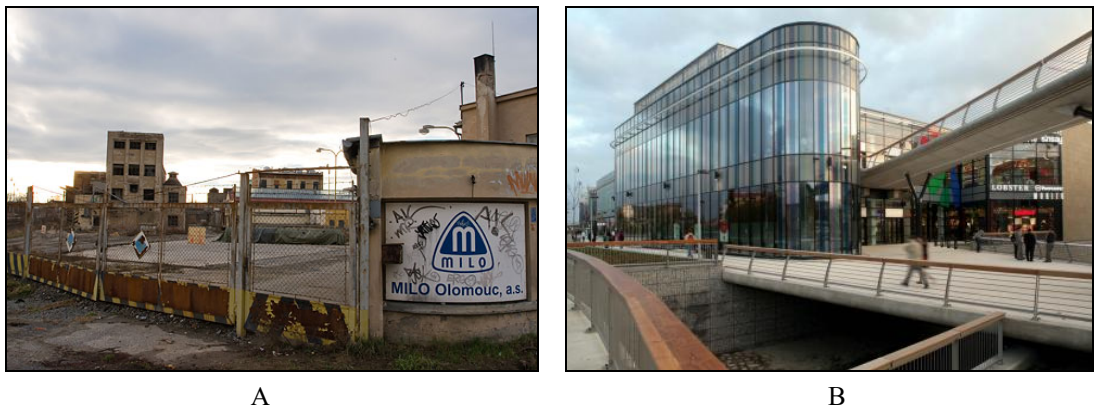
A B Fig. 1: Revitalization of the complex MILO Olomouc a.s., A – the brownfield before the reconstruction, B – the revitalized area OC (shopping centre) Šantovka. (Source: Daniel Mazáč, Metrostav a.s.)
