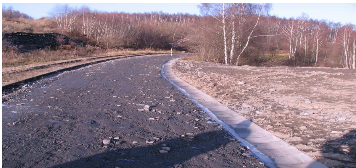
Fig. 5. An example of ground shaping in the Central Heap – ditches [1].
