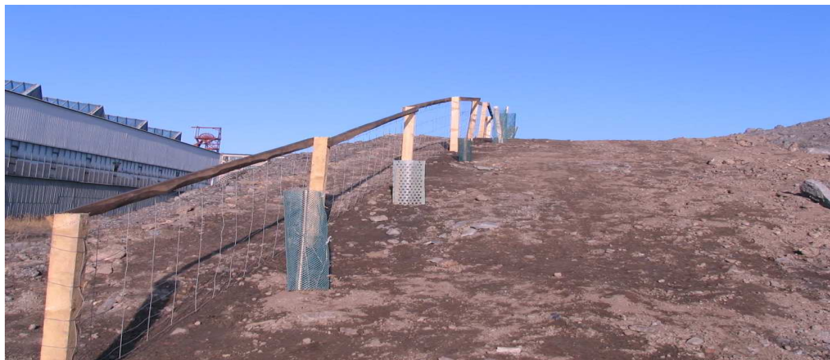
Fig. 7. The geogrid-reinforced structure with a retaining grid and shrub planting [1].
