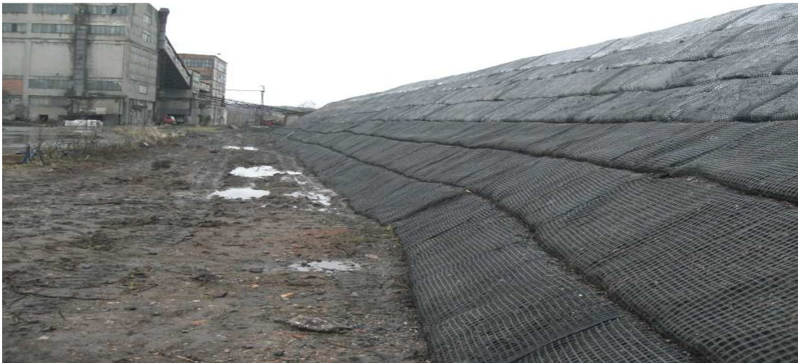
Fig. 2. The geogrid-reinforced structure [1].
