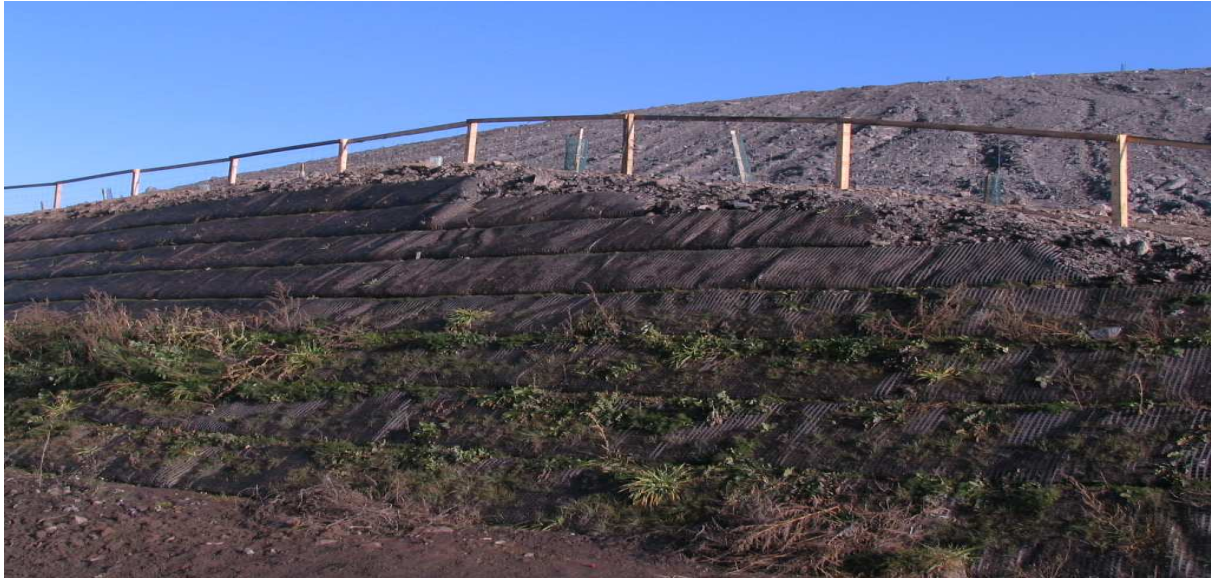
Fig. 6. The geogrid-reinforced structure with a retaining grid and shrub planting [1].
