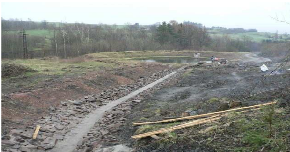
Fig. 8. Ditches are reinforced with stones [1].
