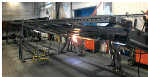
Figure 8 Manual frame welding
