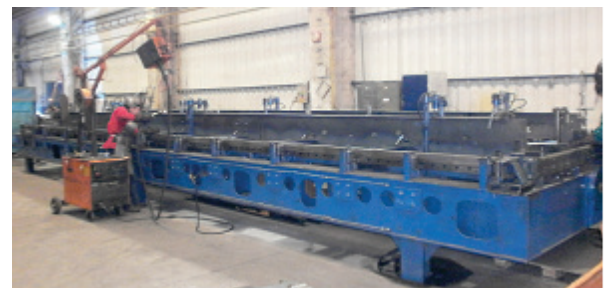
Figure 11 Deck tacking area
