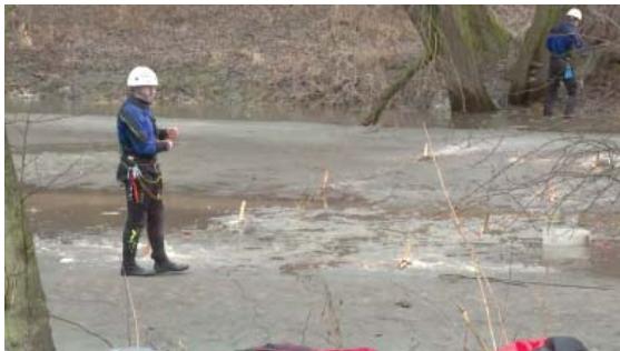
Fig. 5 and 6 The preparation of holes for the placement of charges and the placement of charges beneath the ice surface
