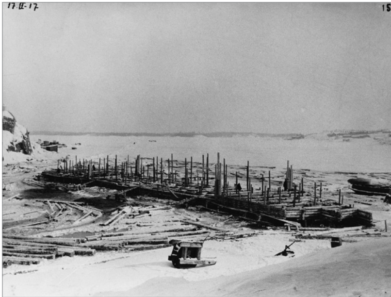
Fig 2.12. The unfinished log barrier embankment (ID 2088) in Tykistölahti ('Artillery Bay') (Photographer unknown/Helsinki City Museum).
