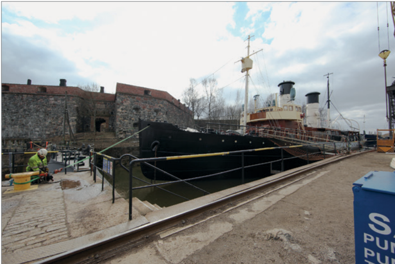
Fig 5.1. The dry dock at Susisaari is still in active use. In the picture icebreaker Tarmo is under renovation. Tarmo serves as a museum at coastal town Kotka (photo by the author 2017).
