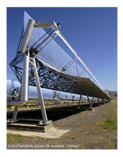
Figure 2.1: ACUREX distributed solar collector field.
