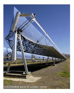
Figure F.1: ACUREX distributed solar collector field.
