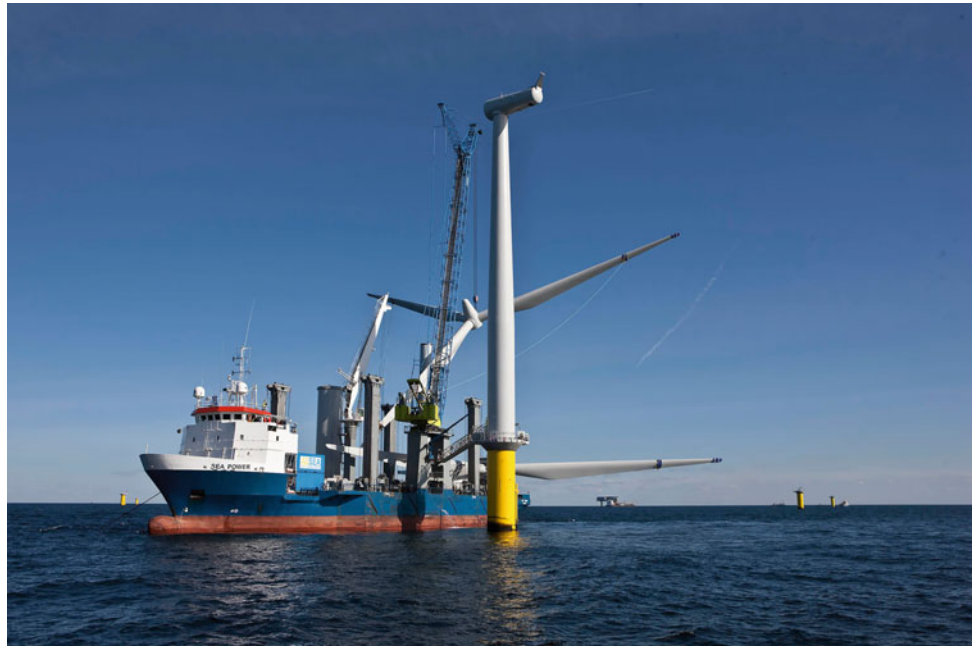
Fig. 14.4 Installation of wind turbine at Horns Rev II wind farm (Picture provided by DONG Energy)
