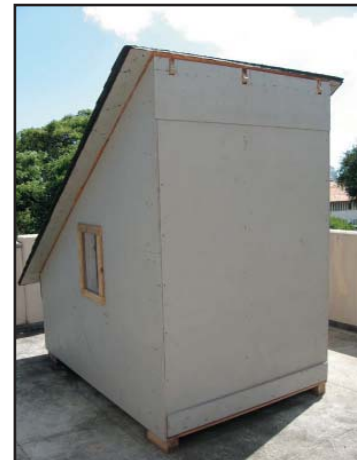
Figure 72: The exterior of Roof Module 3 with the opening for cross ventilation visible.
