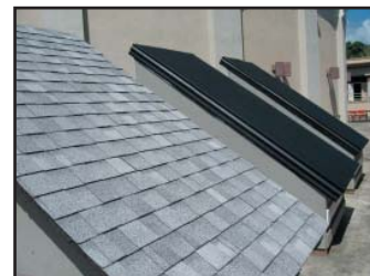
Figure 66: All three roof testing modules located at the University of Hawaii, School of Architecture.
