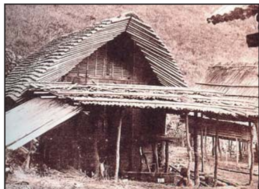
Figure 19: An example of a early structure where the roof and walls are separate components joined together. This particular structure was built by the Isneg tribe. They are known for their boat building skills and the layered bamboo roof mimics the shape of a boat. ( http://www.filipinoheritage.com/images/arts/architecture/early-beginnings2.jpg )
