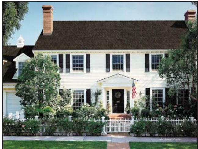
Figure 31: This is a typical asphalt shingle roof on a traditional home in the United States. Asphalt shingles usually last 15-20 years before they need replacement.
