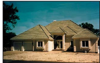
Figure 46: This image shows a typical concrete tile roof. ( http://www.hgroofing.com/images/concrete1.jpg )
