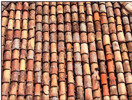
Figure 42: These are Mission or Spanish tiles made of clay and have the same profile alternating facing up and down channeling the water off the roof. ( http://www.digitalapoptosis.com/archives/HR/tile_roof.jpg )
