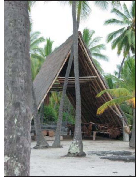
Figure 4: This early Hawaiian structure which sheds water and promotes good air flow is actually nothing but a roof.
