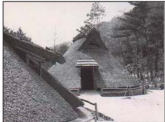
Figure 18: This is an image of a Tateana pit shelter where a pit is dug into the ground and crucks are used to form the roof shape which is covered with thach. ( http://dougukan.jp/archive/tateana.jpg )
