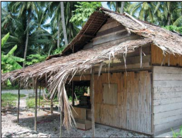
Figure 28 This is an example of a thatch palm roof in a hot-humid tropical climate. The thatching is only 1-2 inches thick and is made of palm fronds. This structure is located in Sumatra, Indonesia.
