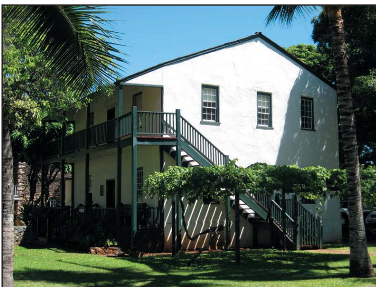
Figure 5: The Baldwin House in Lahaina, Maui is an example of how the Missionaries built structures suited for the colder climates of the northeastern United States in the warm tropical climates of Hawaii. These structures had limited air flow and small roof overhangs causing the buildings to heat due to the solar impacts on the exterior walls.
