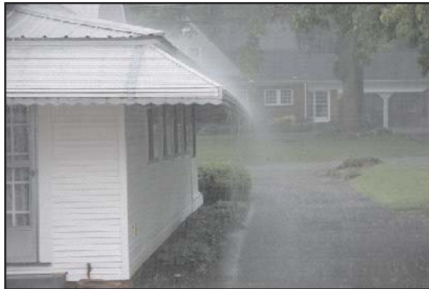
Figure 6: Gravity holds the building on the ground and enables the rain water to be shed off the roof and away from the structure.
