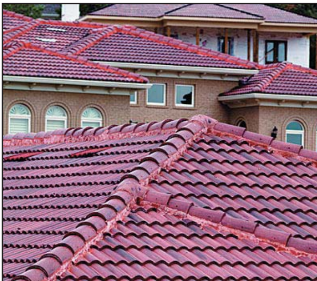
Figure 48 This image shows how a concrete roof can mimic the look of a clay tile roof. The concrete roofs are also less expensive than the clay tile roofs. ( http://www.homeimprovementmag.com/Articles/Images/2006/Mar_roof_concrete.jpg )
