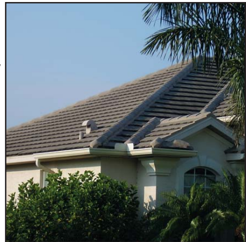
Figure 41: This shows a typical concrete tile roof on a residential structure. ( http://www.bayferrox.com/photo_tour/images/concrete_roofing_tile1.jpg )
