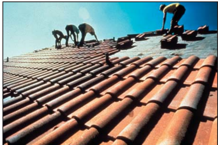
Figure 47: This is a concrete tile roof being installed. ( http://www.concretethinker.com/Content/ImageLib/pcano5079.jpg )
