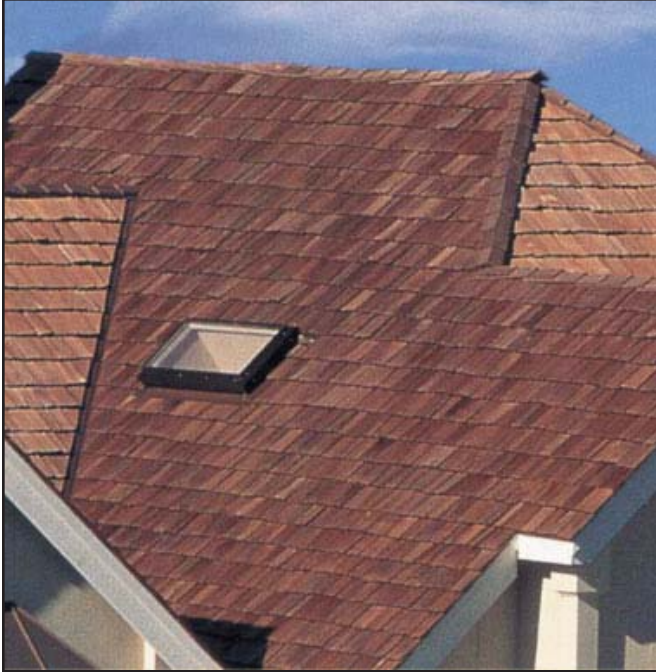
Figure 36: A wood shake roof is one of the most attractive roof coverings, but their high cost keeps many homeowners from installing them.
