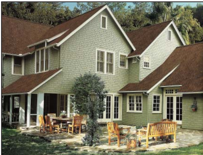
Figure 32: Asphalt shingles come in a wide variety of shapes and colors which are fairly inexpensive as compared to other roofing materials. They can be applied over all types of roof designs by any contractor or handyman.
