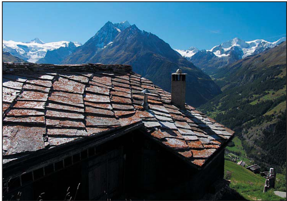
Figure 40: The slate shingles on this roof are huge. They must be at least 2'x2' if not larger. This is an old slate roof dating back well over one hundred years. ( http://www.photoseek.com/05ALP_3303-Arolla-Valley-slate-roof.jpg )
