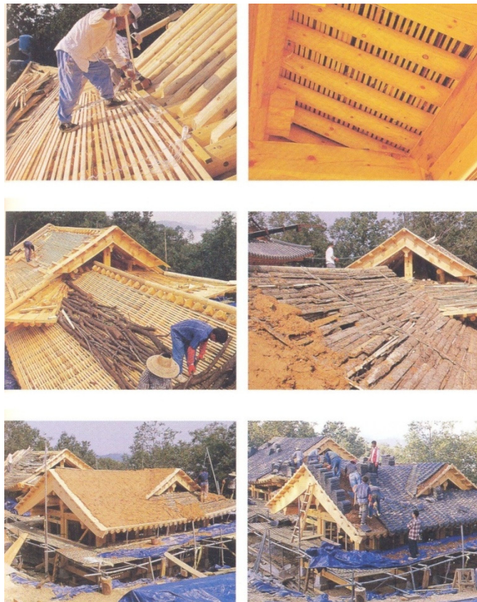
Figure 2-4 Roof construction, it provide the roof thickness about 30 centimeter ( (D. K. Kim 2004)
