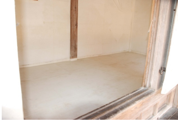
Figure 2-5 Yeongyeongdang Windows, the inside windows are sliding type and outside windows are swing door.
