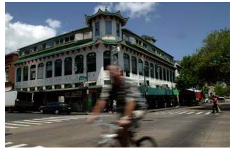
Figure 34 Wo Fat Building
