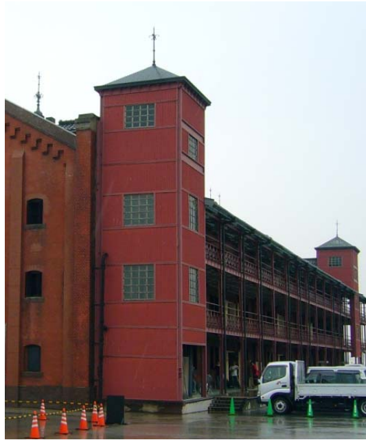
Figure 11. Here is an example of superimposed work. Yokohama Red Brick Warehouse's construction was completed in 1912. However, the original elevator shaft and machinery was later added to the Yokohama Red Brick Warehouses in 1956, by the Yokohama City Customs Administration of the time. 14 But because the exterior metal trellis has become part of the building's character, rather than restoring the original look, the architectural designer has restored the elevator and exterior trellis. Source: Author, 2008
