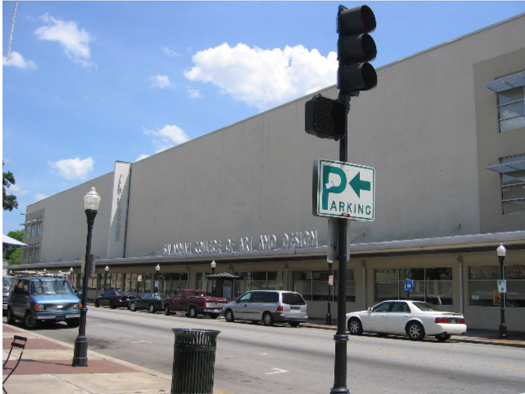
Figure 59. The Jen Library at the Savannah College of Art and Design is an example of Middle American adaptive reuse of big box buildings of yesteryear. The Jen Library building, open to the public and students, was once 85,000 sq. ft unspecified department store. Source:
