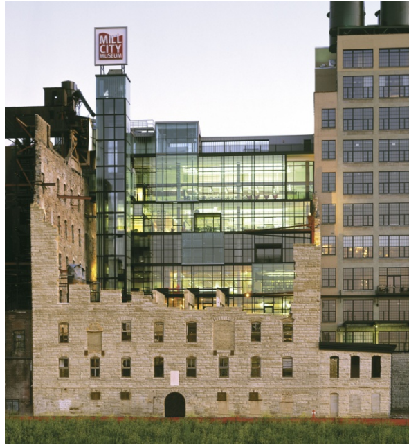
Figure 14. The adaptive reuse of the Mill City Museum in Minneapolis deliberately exudes patina by maintaining the post-explosion walls as they were, using them as an element that reflects the building's character. It also serves as a barrier from the outside into a courtyard. Source: http://events.mnhs.org/media/Images/Sites/mcm/MM_300.jpg , 2010.
