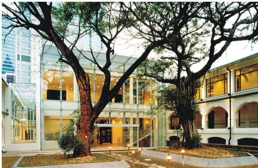
Figure 32. The Whitfield Barracks, now the Hong Kong Discover Heritage Center, utilizes new facilities (elevator and lobby on left) that are separate from the original barracks (on right).
