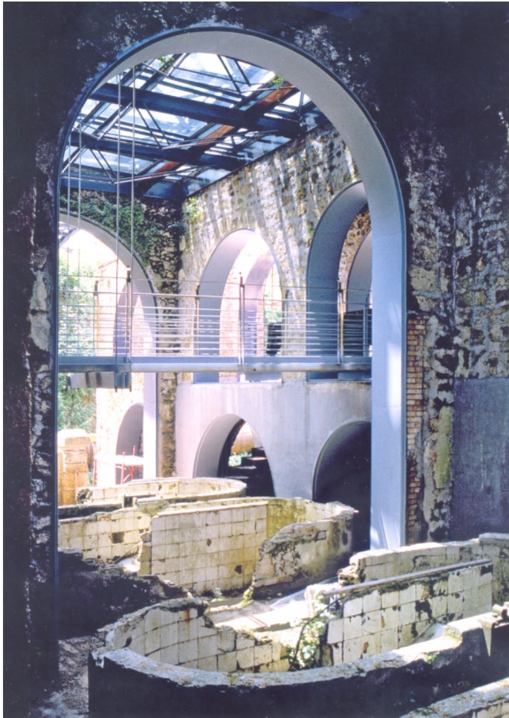
Figure 33. Gangways and walkways can relieve stress on existing building. Source: Source: Old Buildings looking for New Use by Pierre Thiebaut.
