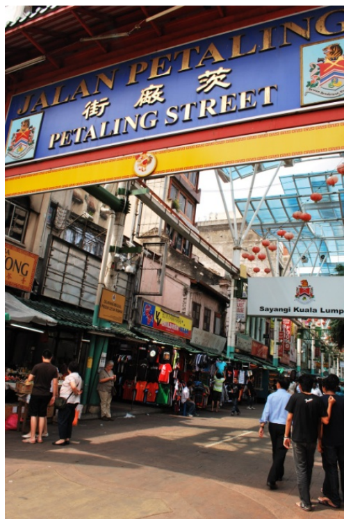
Figure 63. As a gathering place, Petaling Street is a successful magnet for social activity, despite its poor reuse of architecture. From this view, traces of the original architecture façade poke through the modern signage. Source: http://ketchuptomyfries.blogspot.com/2009/11/petaling-street.html
