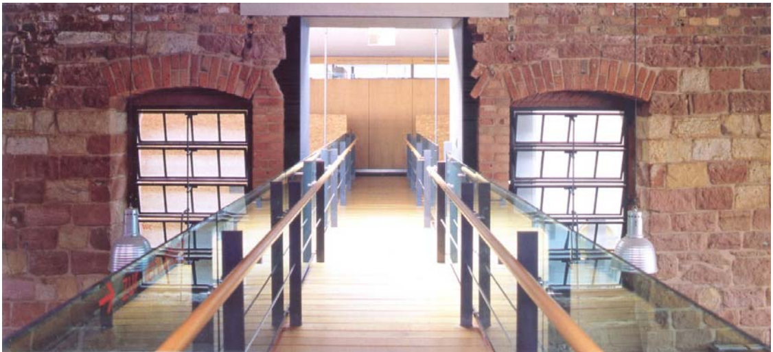
Figure 29. A contemporary bridge at the Stadtbibliothek in Landau, Germany permeates the existing abattoir building façade, and links the contemporary offices with the reading rooms. Source: Old Buildings looking for New Use by Pierre Thiebaut.
