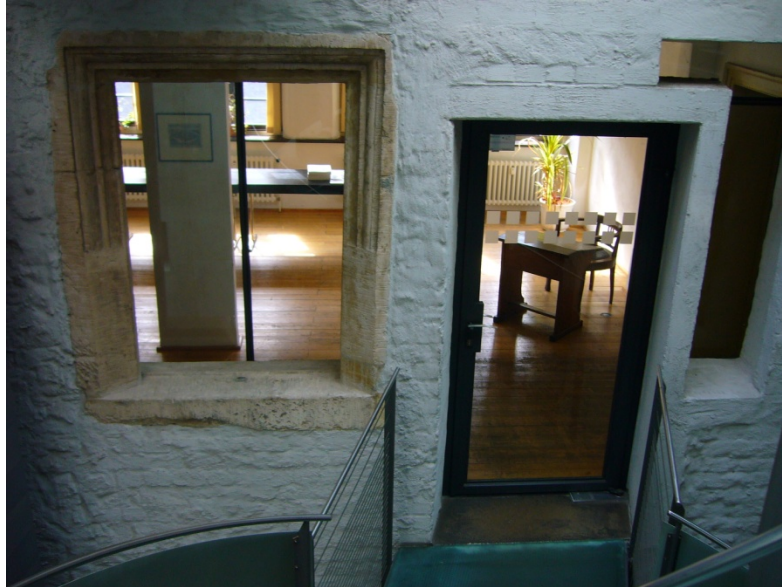
Figure 5. The Alte Nikolaischule's installation creatively ignores the boundaries of preexisting window borders to fabricate doorways that are muted. Next to the doorway, the window orifice retains its original stone material, albeit with minor wear. Source: Author, 2010
