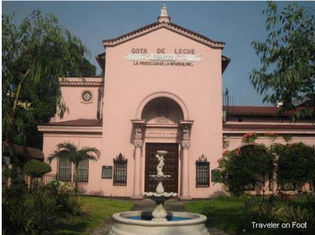
Figure 52. Once a forgotten building of Italian renaissance style, the Gota de Leche redevelopment and subsequent award for restoration by UNESCO in 2003 spearheaded the idea of viability in restoration. Source: http://traveleronfoot.wordpress.com/2008/02/17/gota-de-leche/
