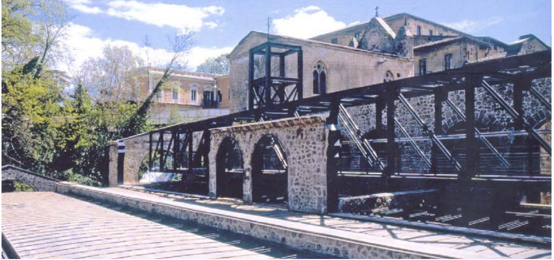
Figure 28. The Museo della Carta, located in Isola del Liri, Italy, was once a cardboard factory, and before that was once a convent. Here, the construction of a entrance footbridge, with a partial archway, shows an intense relationship of old with the new blackened metal structure. Source: Old Buildings looking for New Use by Pierre Thiebaut.
