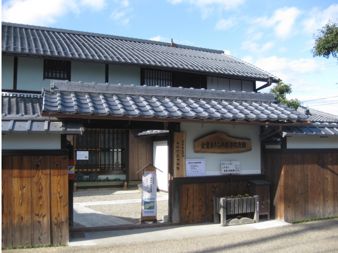
Figure 64. An example of a Machi-nami building in Gokasyu Town, Japan. The front door of the building, which is coincidentally the Center for Machi-nami Preservation, is stepped up and is clearly an ADA violation – if the building were to be reused in an American context. Source: http://upload.wikimedia.org/wikipedia/commons/e/ee/Kondo_machinami_hozon_koryukan.JPG
