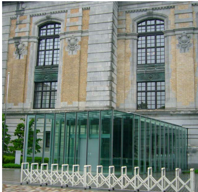
Figure 17. Sometimes, the confines of the existing building cannot fit the function of a lobby, and a addition for a lobby must be made like The Children's Library at Ueno Park, Japan. Source: Author, 2006.
