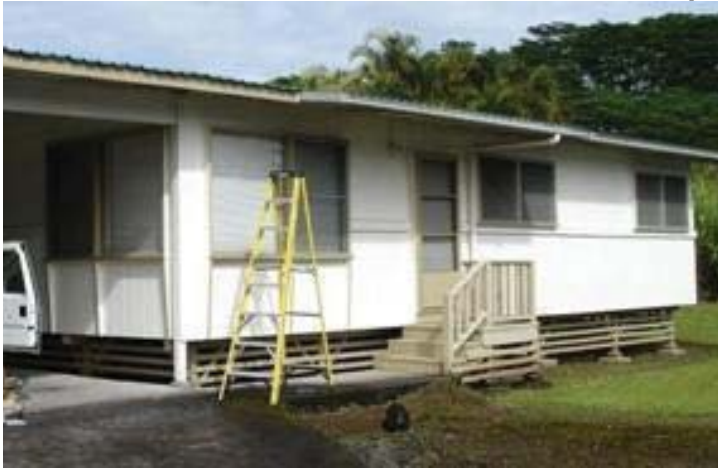
Single wall construction typical of older homes in Hawaii
