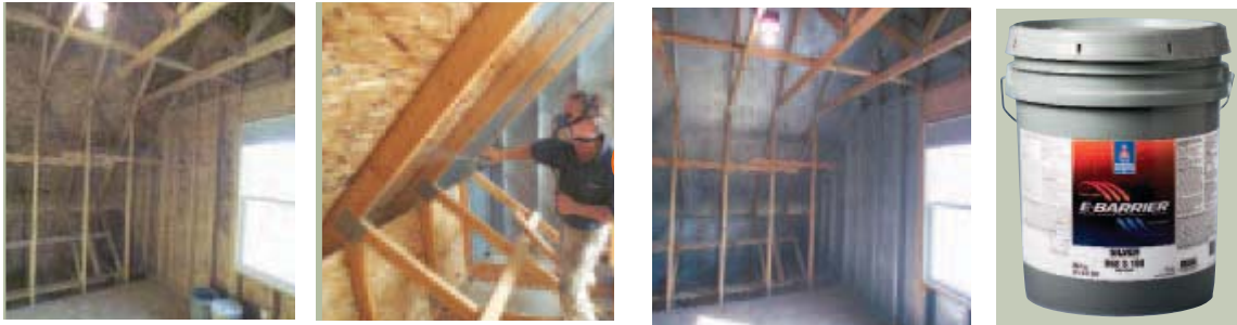
E-Barrier being painted onto attic surfaces
