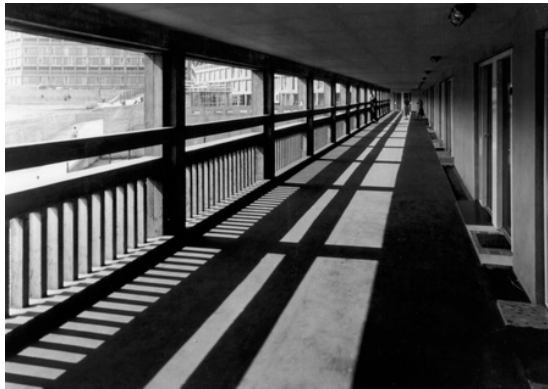
Figure 25: Exposed concrete single loaded
