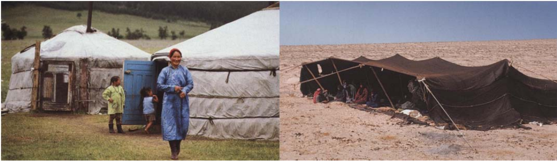
Figure 14 (Left) A family outside of a yurt found in Mongolia. The retractable framework that creates a diamond design is covered by felt. (Right) The Bedouin black tent is a tensile structure that is constructed of woven goat hair fabric, ropes and poles.
